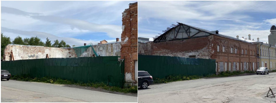
Figure 4.26. Current status of the structure (Tomilina, Gontar, & Frolova, 2020).
