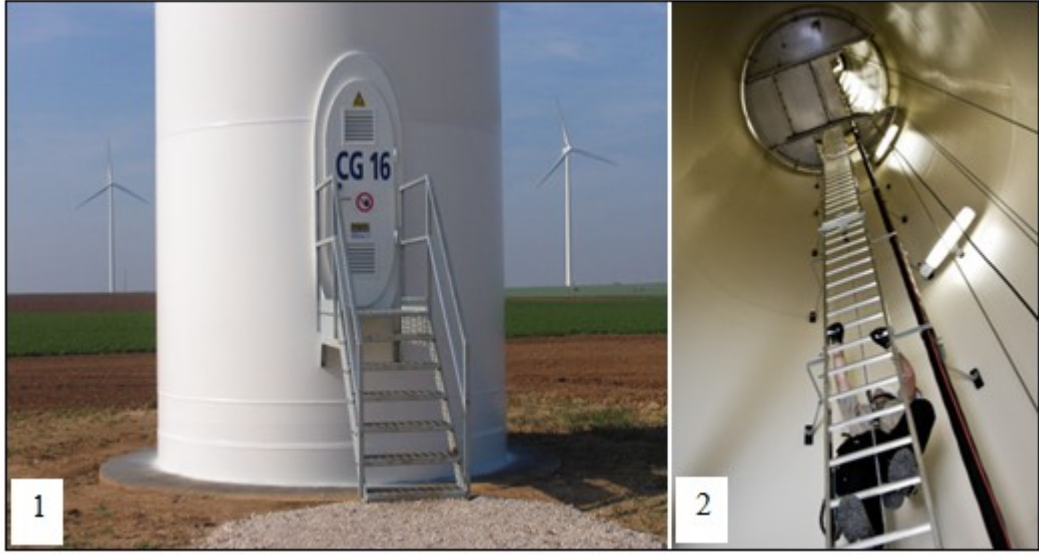
Şekil 2.6. Kule giriş kapısı ve kule içi güvenlik merdiveni (1. http://www.freshford-somerset.co.uk/cutenews/data/upimages/windturbinedoorway.jpg , 2011 ; 2. http://www.gravitec.com/training/fall-protection-rescue-training/wind-turbine-climber-rescue-competent-trainer-refresher.html , 2011)
